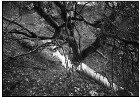
COURTESY OF MARK MOSLEY Storm waters have carved an artificial ravine that is 30 feet deep and 70 feet wide and endangering neighboring houses.
